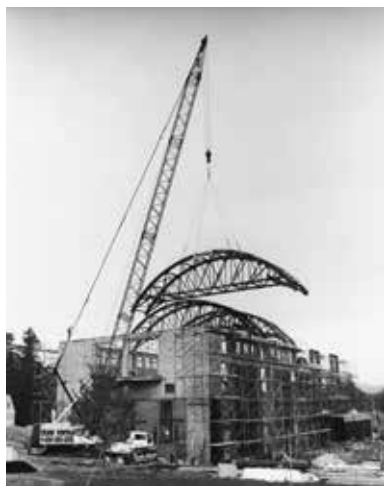
The lowering by crane of a steel arch to form the roof of Seiji Ozawa Hall, 1993 (Walter H. Scott)
